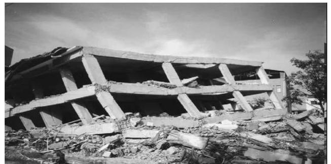
**Figure 1:** Beam column Joint fails due to shear failure in Kocaeli Earthquake
