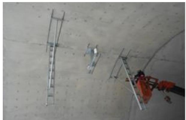
Figure 2: The work of attaching some steel parts in the tunnel
