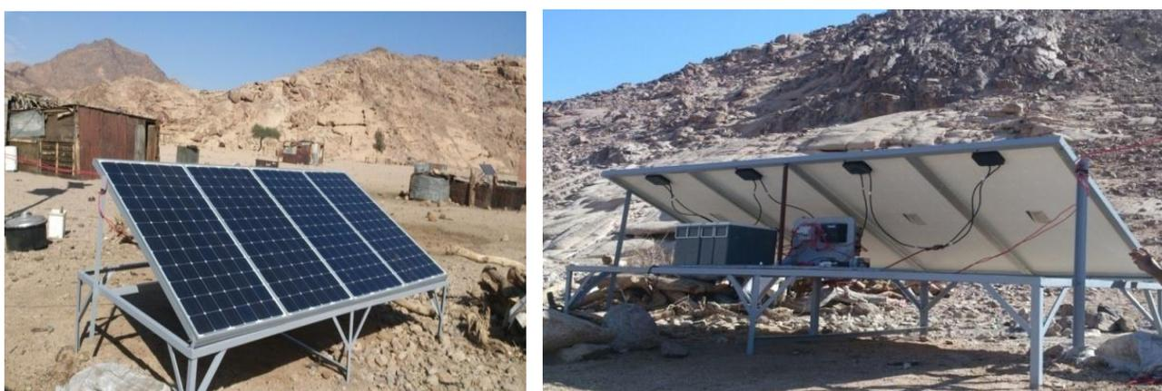
**Figure 12:** Installed stand-alone PV system.
