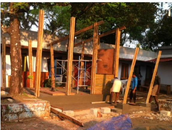
**Figure 13:** Use of locally available bamboo for construction of the canteen
