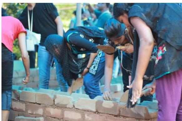
**Figure 5:** Laying of the CSEB Masonry as a ‘hands on’ built exercise
