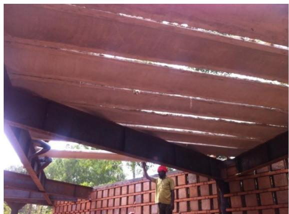
**Figure 11:** Use of light weight Ferro cement Shell placed between the steel members
