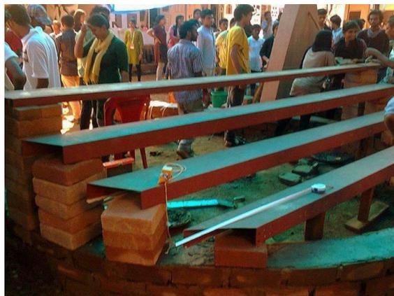
**Figure 6:** Use of discarded electrical trenches as seating
