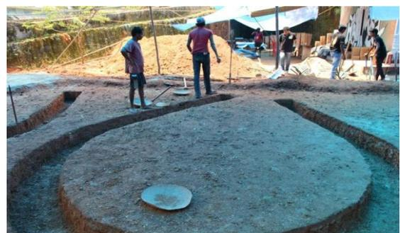
**Figure 3:** Using Rammed Earth Foundation for the Amphitheatre.
