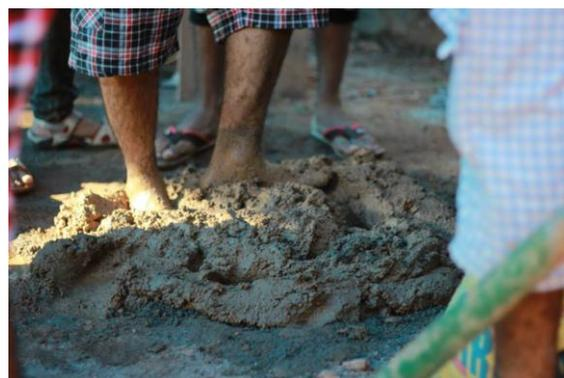
**Figure 7:** The making of Earth plaster for the structure
