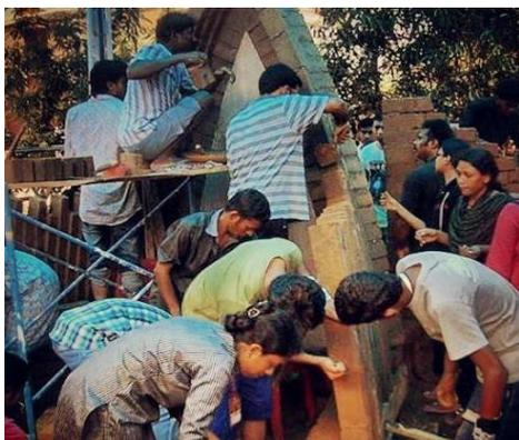
**Figure 4:** Construction of the Nubian Vault by the students as Shading structure in the design of the Amphitheatre
