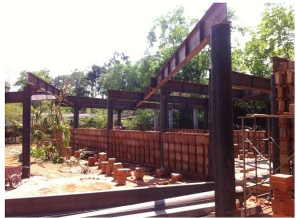
**Figure 10:** Structure built using steel sourced from the local shipyard
