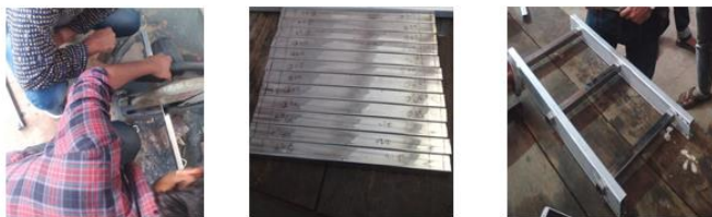
Figure 5. fabrication of ladder frame
