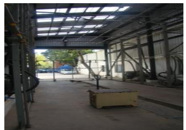
Figure 3. Structure enclosure at rain test chamber.
