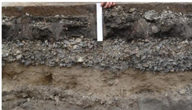
**Figure 4.** The example of road base operated structure on highway M-4 “Don”.
