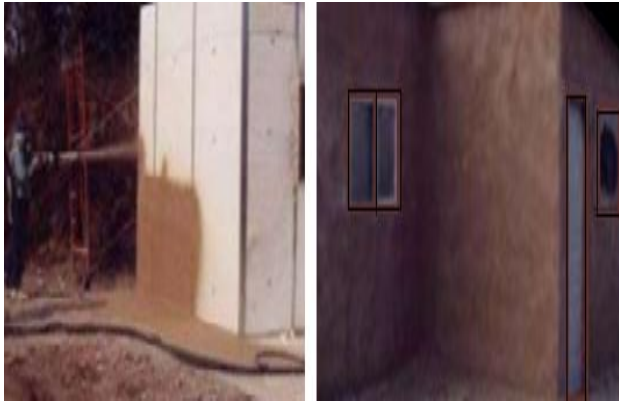
Figure 3. Spraying the grancrete mixture
