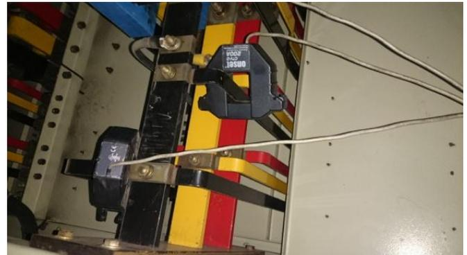
**Figure 5.** Power meter (Black with Wire) is Clamped on Electricity Panel
