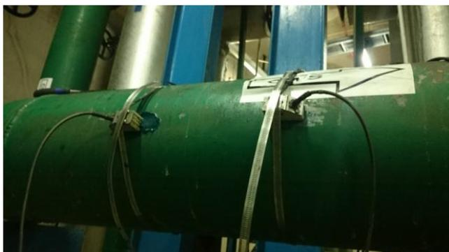
**Figure 4.** Flow meter Ultrasonic (Transmitter and Receiver) placed on the Pipe
