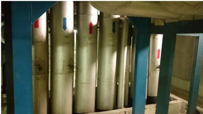
**Figure 2.** Chilled Water Pipe (Supply and Return)
