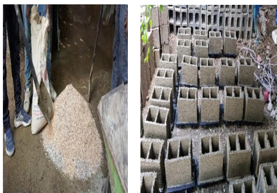
Figure 1. Dust plywood mixing and placing of HCB
