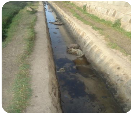
Fig. 8: Semi-Closed Drain, Picture Credit by Author, 2015
