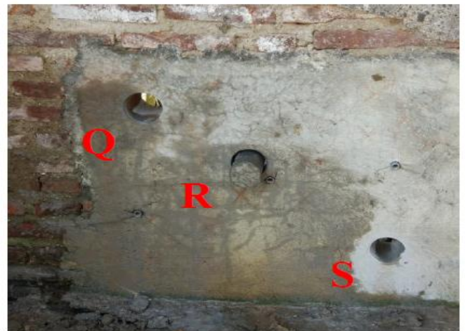
Fig 11. Core Drill sampling of retrofitted masonry wall
