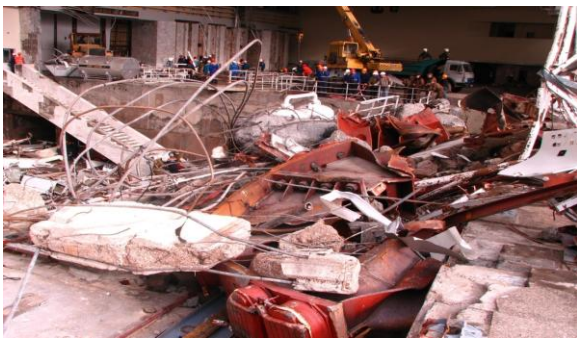
Fig.2 Sayano-Shushenskaya Hydroelectric Power Plant accident caused by a failure of the automated system for process monitoring and control
