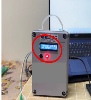
Figure 8. Real-time current reading and PD status displayed on the Arduino monitoring unit
