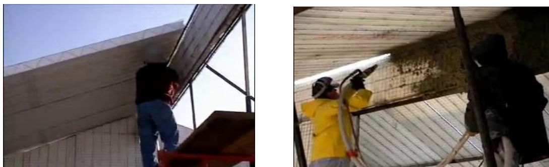
Figure 5: Figure showing the assembling of roof and concreting
