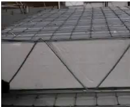
Figure 4: Cross-section of EPSCSR before concreting [3]
