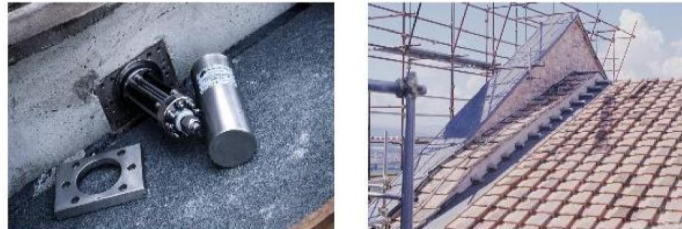
Fig. 6: SMA Devices in the Basilica of St Francesco of Assisi [Castellano et al., 2000].
