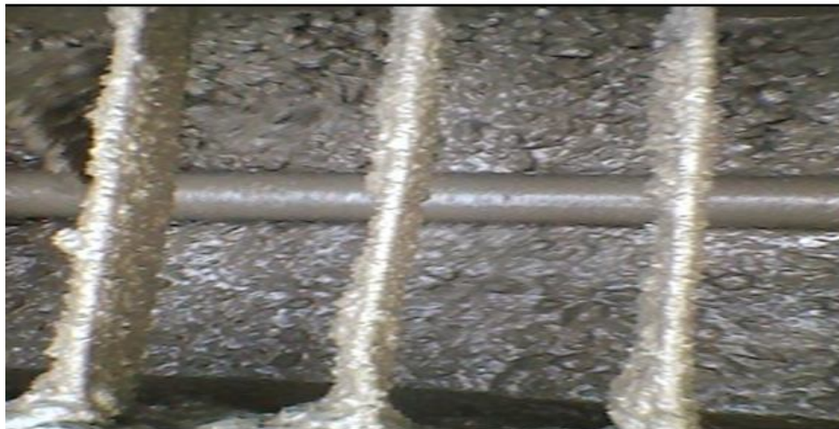
Fig. 2: GBS& CSS blended concrete in pump hopper.
