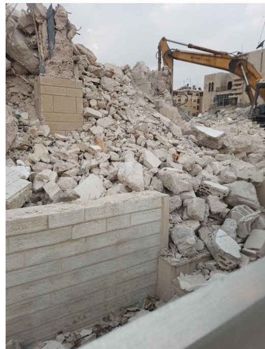
Figure 1. A location for demolition in Amman
