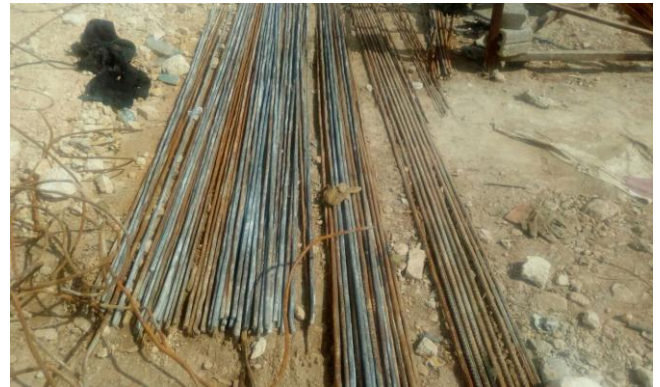
Figure 5. Sorting of steel bars
