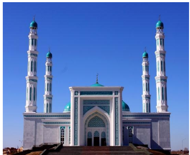
Fig. 3. A general view of the Karaganda mosque
