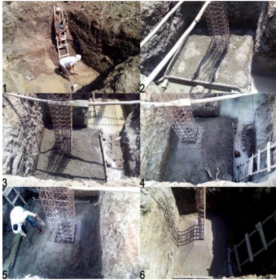
Image 2: Sequence of foundation casting on site.
