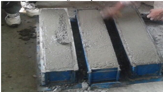
Fig.6 Casting of beams
