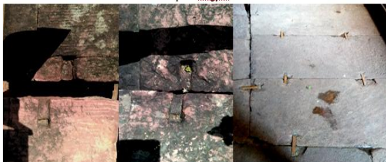
Evidences of Similarity in Plinths as well as in Joinery of Stones of Temples at Ashapuri and Shiva Temple at Bhojpur
